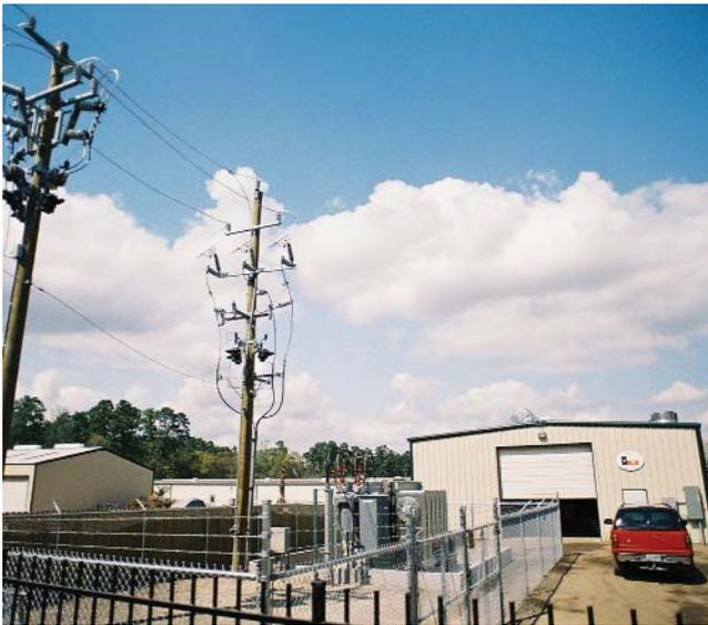
This substation, located outside of Biofuels Power, converts electricity produced by Biofuels Power from medium-to high-voltage so it can be connected to the electrical grid and distributed on a high-tension distribution voltage line.
