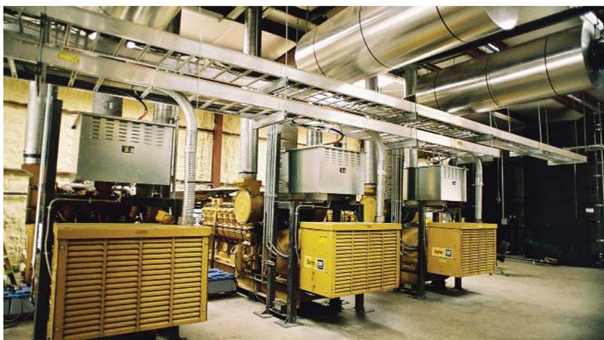
Biofuels Power can produce up to 5 megawatts of electricity using these three Caterpillar generators that run exclusively on biodiesel produced by Safe Renewables.
