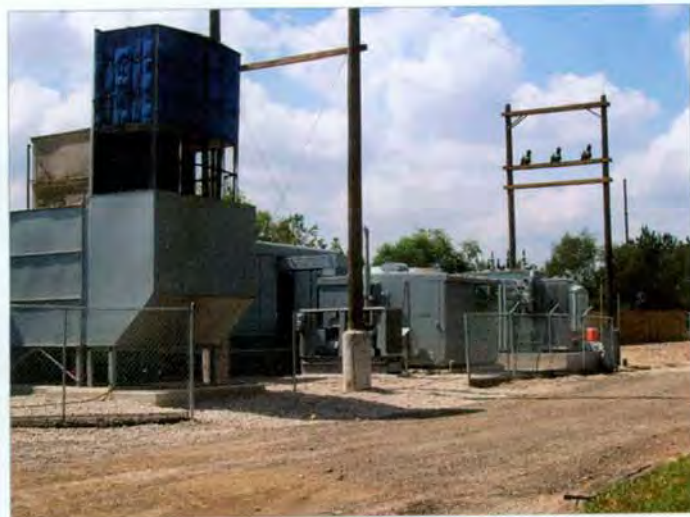
Biofuels Power's 10 MW GE Frame 5 turbine can operate on biodiesel that doesn't meet the ASTM specifications. This gives the company access to lower cost fuels.
